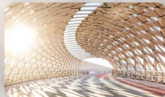
Atyrau Bridge Astana
